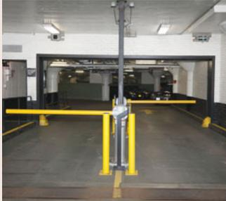
4 All six indoor parking facilities utilize HID card readers and parking gates. The integrated system provides access control and validation for billing purposes for a third-party operator.
