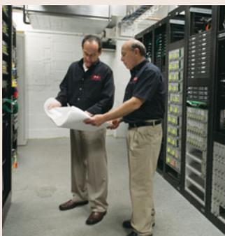
1 SMS project engineers review schematics at one of five security hubs. Each room is equipped with APC UPS backup power, Verint camera encoders, video servers and video storage, in support of about 20 buildings and the residences.
